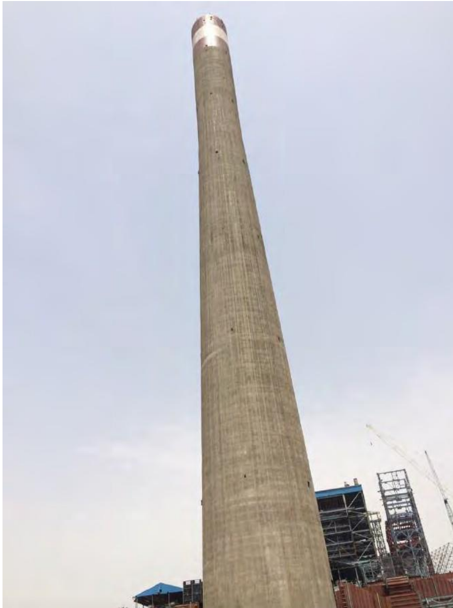
275 Meters RCC Chimney Works of Unit#3 at 3 x 660 MW Bara Thermal Power Plant, Shankargarh, District- Allahabad, Uttar Pradesh.
